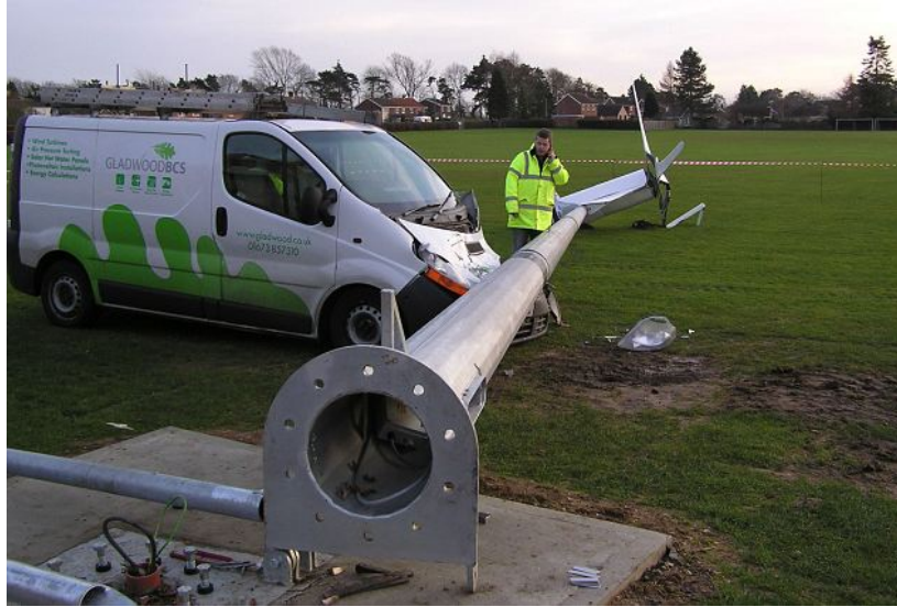
Figure 4. Wind turbine 40-ft tower collapse while being mounted at the playing field of the Fakenham High School, Norfolk, UK, 2009.
