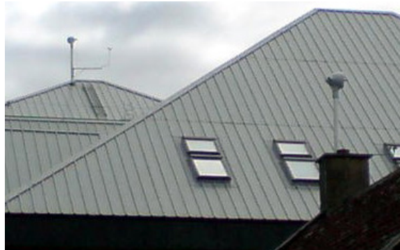
Figure 6. Roof wind turbines removed for repair.
