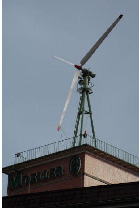
Figure 2. Tied down rotor on an inoperational Allgauer derivative wind turbine on top of a building at Holzhausen, Rheinland-Pfalz, 2005.
