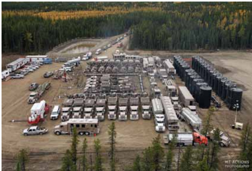
Hydraulic fracture stimulations for shale gas or tight gas reservoirs often require large amounts of equipment on site during the treatment operations
